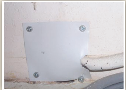
Power supply hole sealed with metal flashing.*
