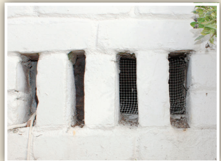
Check for loose mesh in foundation vents.
